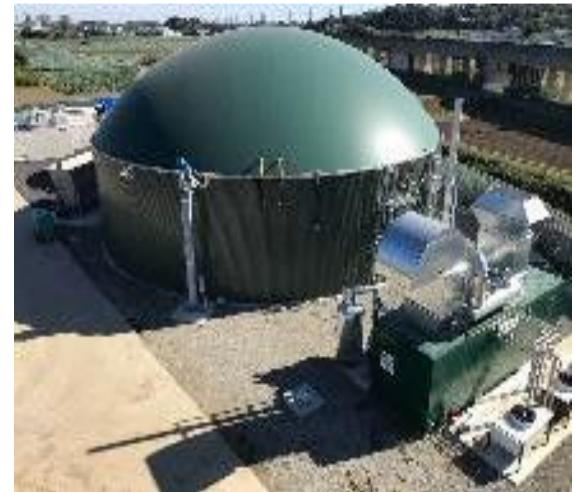
□ Anaerobic digestion (AD) systems are designed to capture the biogas produced from this breakdown and produce energy. AD’s place on EPA’s Waste Management Hierarchy depends upon the final disposition of the digestate. If the digestate is beneficially reused (e.g. composting, land application), AD would reside in the “Recycling/Composting” category. If the digestate is ultimately landfilled however, AD would reside in the “Energy Recovery” category.
